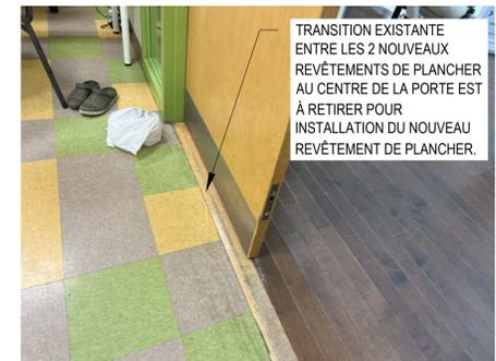
TRANSITION EXISTANTE ENTRE LES 2 NOUVEAUX REVÊTEMENTS DE PLANCHER AU CENTRE DE LA PORTE EST À RETIRER POUR INSTALLATION DU NOUVEAU REVÊTEMENT DE PLANCHER.
